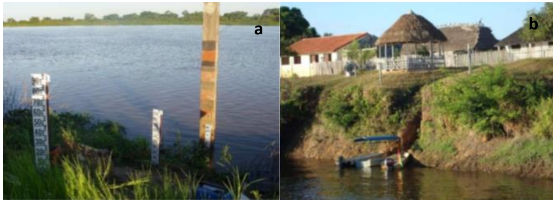
Figure 3. Types of hydrometric stations: a) sectioned staff gauge limnimeter in Puerto Busch, Rio Paraguay, b) Top level bank reference limnimeter at Versailles, Itenez River. Source SNHN.
